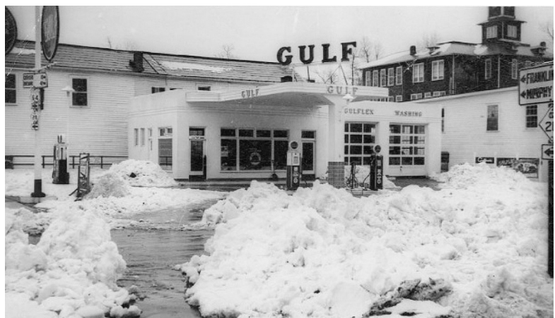
Had to plow a path to get to Bryson's Gulf Station!
